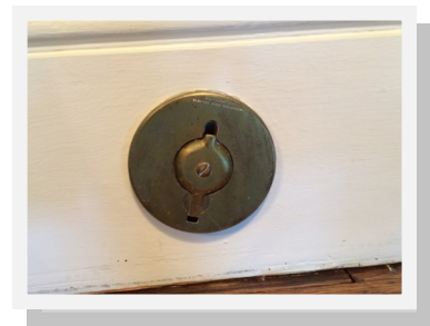
This outlet provided a place to insert a central vacuum hose.
